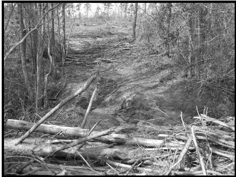
Figure 1. Shows slash being utilized on the approaches of a closed out stream crossing. Slash can be an excellent erosion control tool for stream crossings; however, just make sure slash is minimized from being placed in the streambed.
