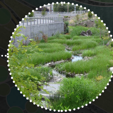
Green Storm Water Infrastructure
