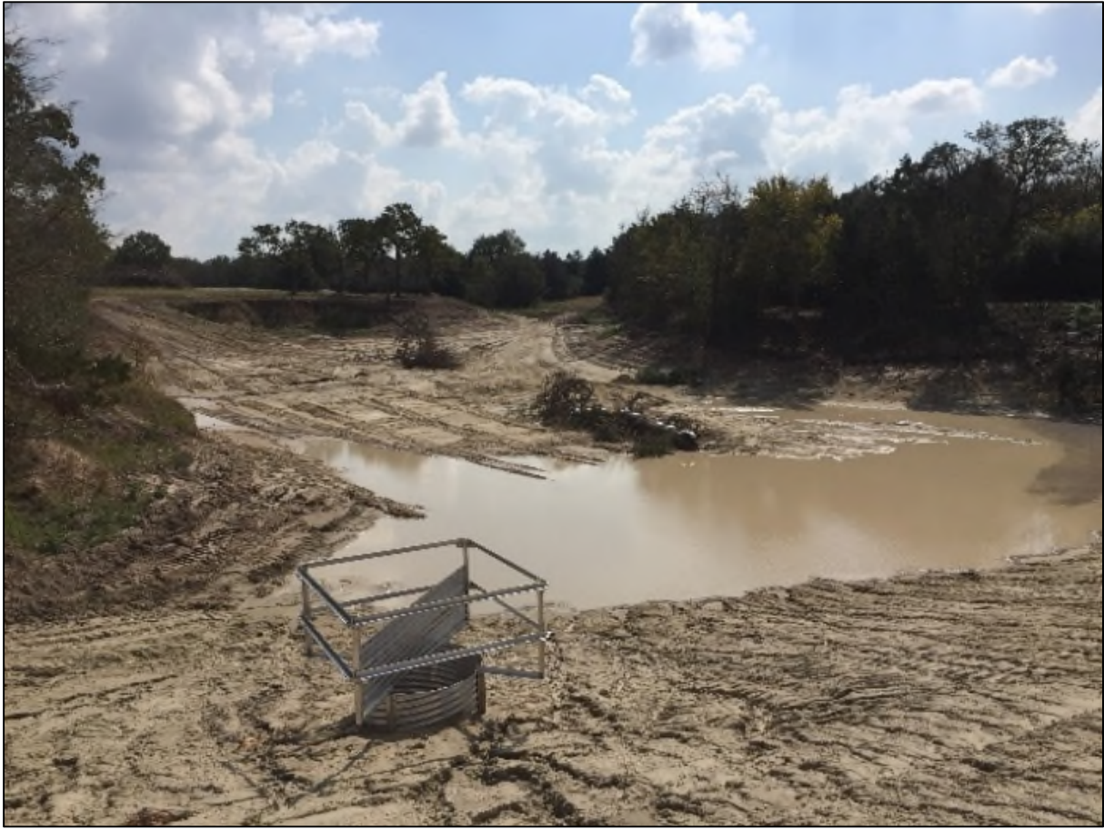
Photo 5: Another grade stabilization structure installed by Dr. Russel Clark of Fayette County. Not only did this structure help reduce erosion and sedimentation, but also created an alternative water supply for livestock.
