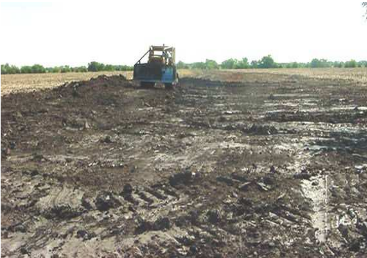
The waterway above is staked and reconstructed
