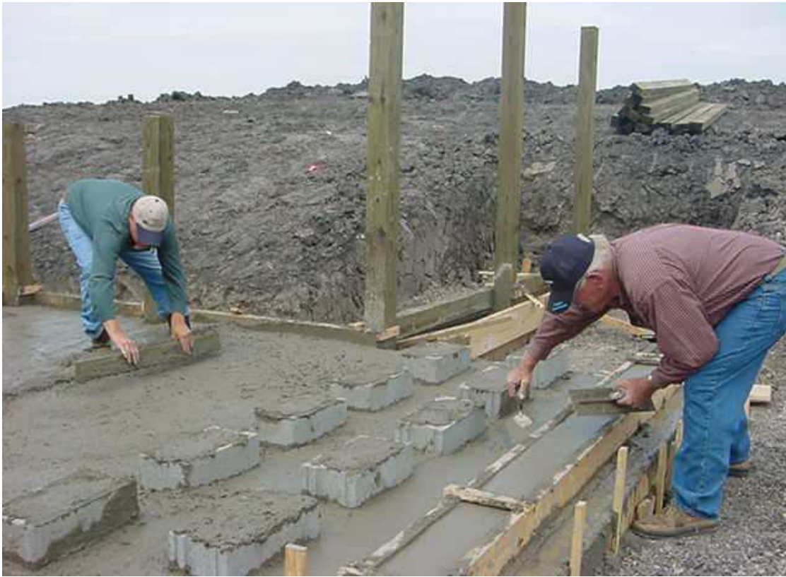
Construction details showing foundation forms being filled with wet concrete and the cured concrete ready for the form removal. (Below)
