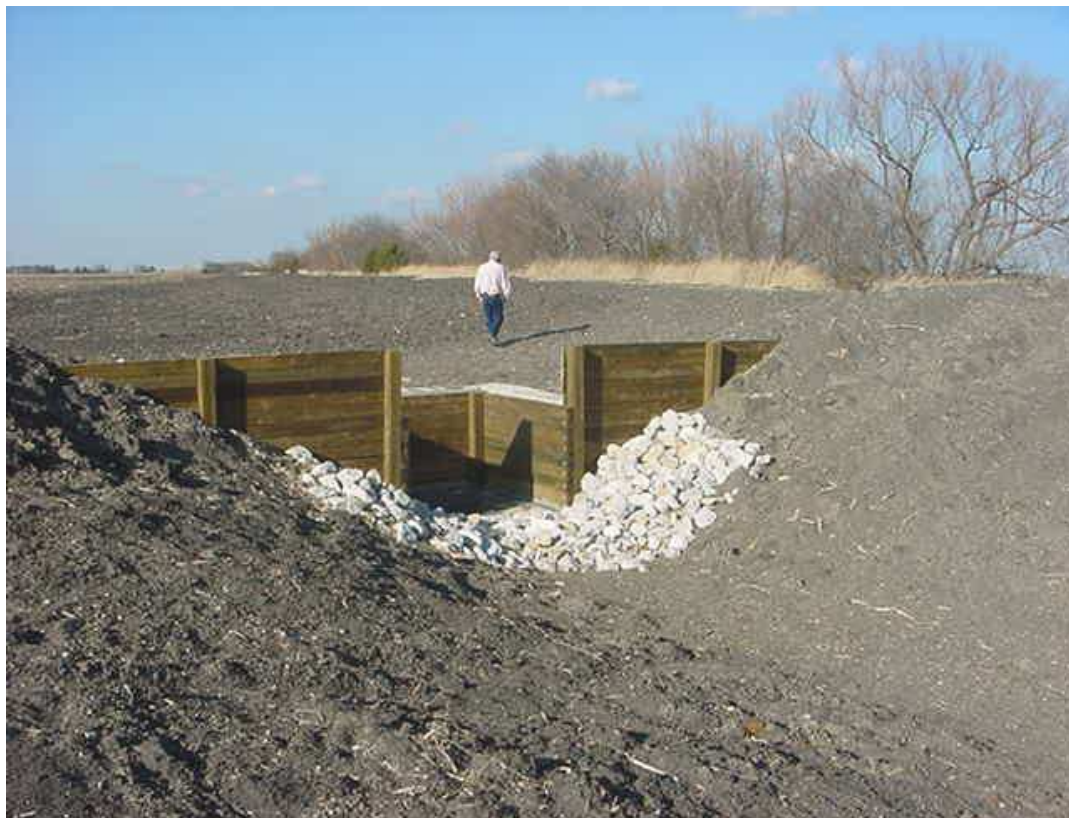
Compaction of the soil is needed to prevent excessive settling around the walls. A completed toewall with rock riprap to control erosion at site of water discharge is shown below.
