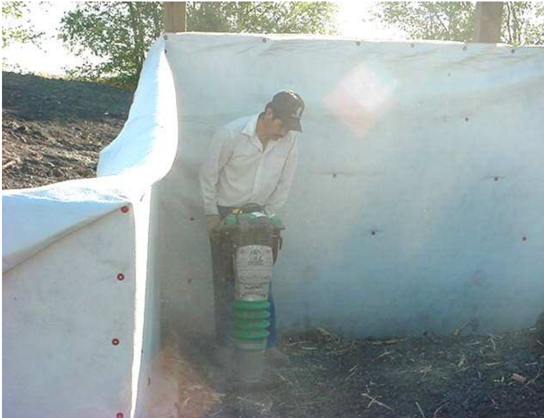
Compaction of the soil is needed to prevent excessive settling around the walls. A completed toewall with rock riprap to control erosion at site of water discharge is shown below.
