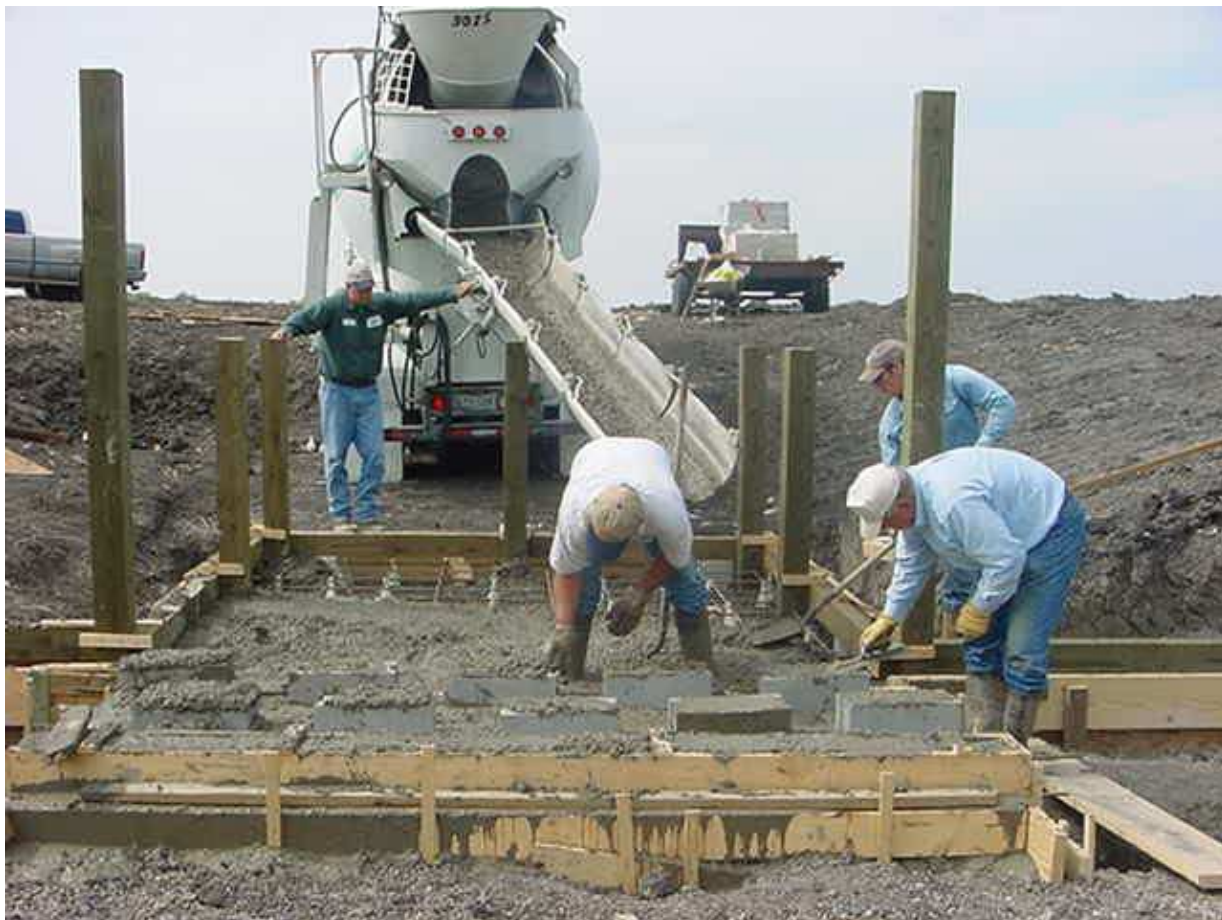
A wood toewall is constructed near the end of the of the waterway to provide four feet of vertical drop for the discharged water
