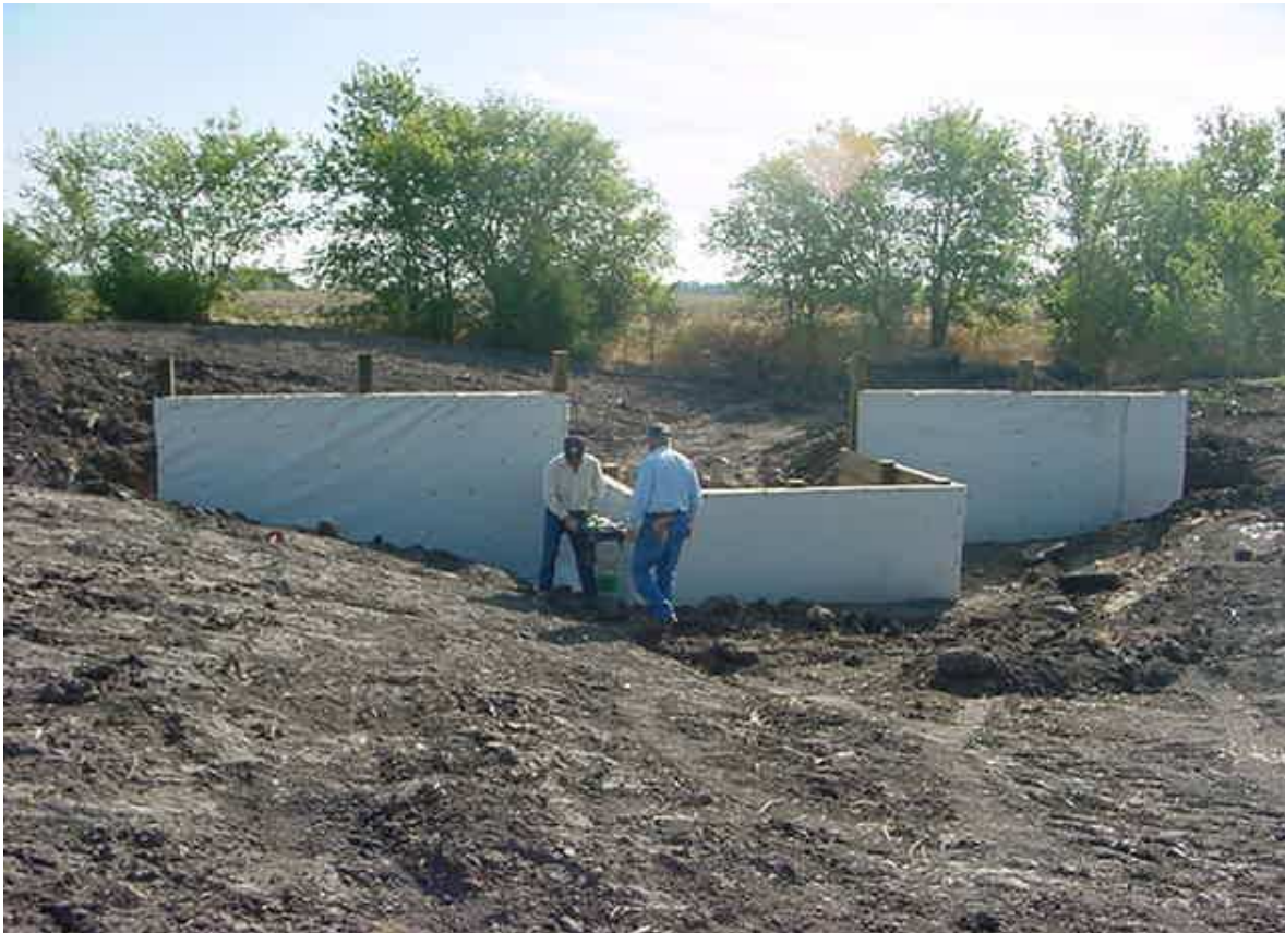
A wood toewall is constructed near the end of the of the waterway to provide four feet of vertical drop for the discharged water
