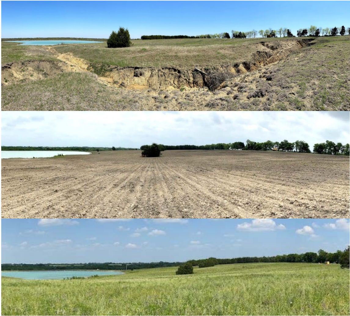
Figure 6. Severe case of classic gully erosion (top) which was reshaped by heavy grading and sprigged to bermudagrass (middle). Recovery of this field was further supported by applying cover crop with the assistance of NRCS (bottom).
