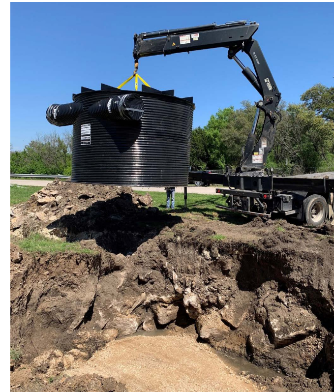
FIGURE 2.5 Installing the vortex separator (Photo by UCRA)
